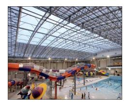
Natural light and illumination Traditional construction simply doesn't allow as much natural light. OpenAire roof and sidewall glazing options include glass, polycarbonate and EFTE. An OpenAire roof creates an exceptionally bright and spacious environment.
