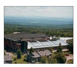
Natural ventilation With a retractable roof enclosure, an opened enclosure produces natural ventilation, which substantially reduces a waterpark operator's reliance on running a mechanical system for dehumidification and ventilation. This reduced reliance on mechanical ventilation generates substantial energy savings in the long-term.
