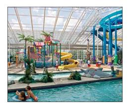
Maintenance free Unlike steel framing, OpenAire's maintenance-free, thermally broken aluminum framing system stands up to moist, chemical aquatic atmospheres and never needs to be repainted.
