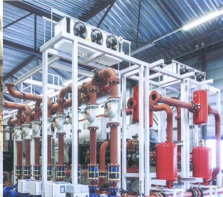
Example skid mounted pre-fab plant room installation for an Unlimited Snow facility
