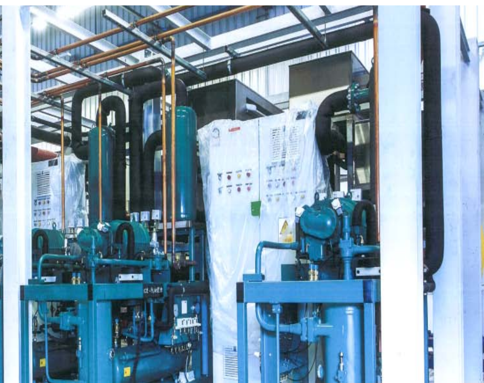
Example skid mounted pre-fab plant room installation for an Unlimited Snow facility
