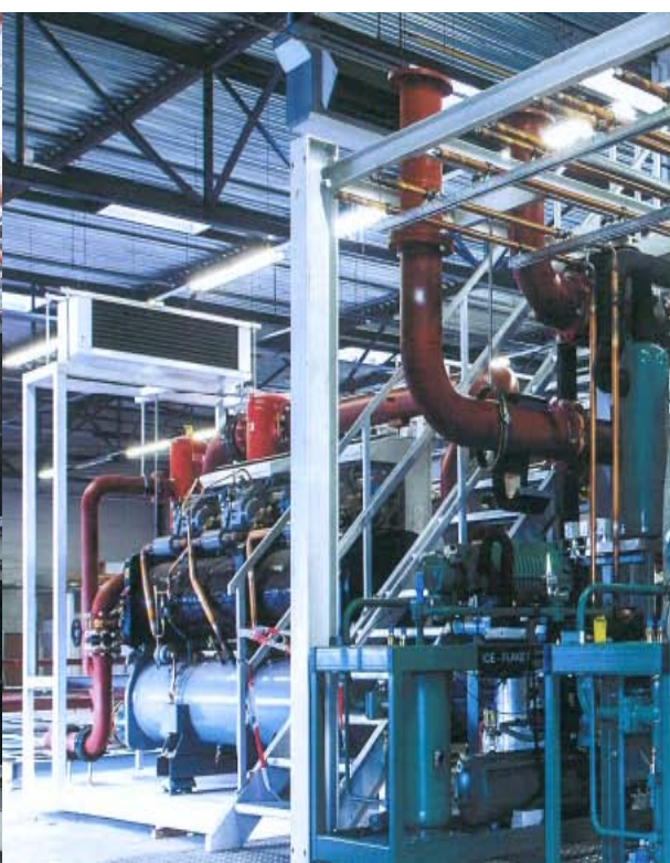
Example skid mounted pre-fab plant room installation for an Unlimited Snow facility
