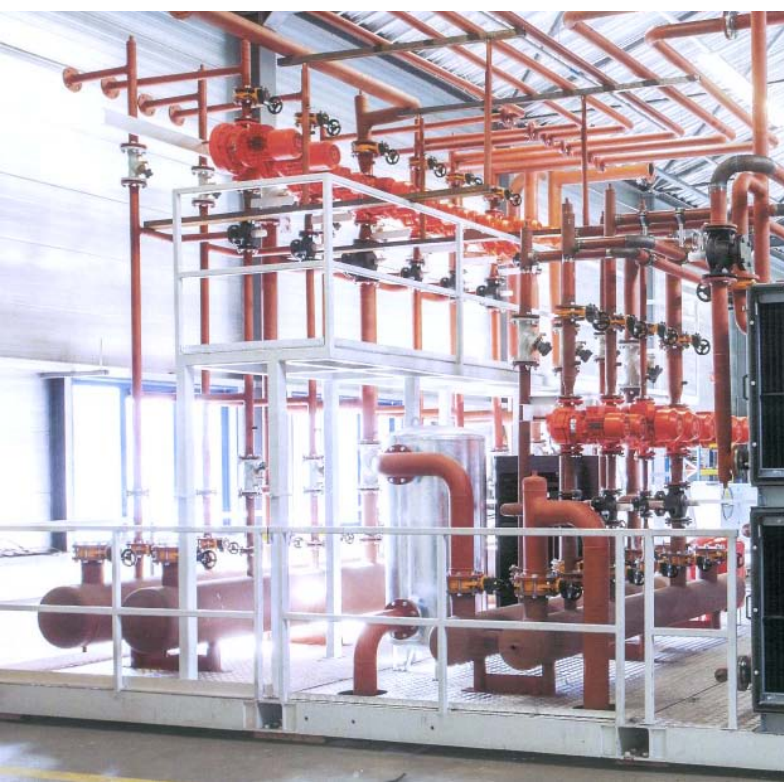
Example skid mounted pre-fab plant room installation for an Unlimited Snow facility
