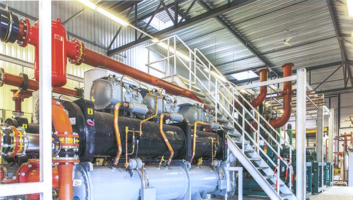
Example skid mounted pre-fab plant room installation for an Unlimited Snow facility
