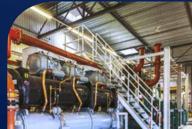
AN EXAMPLE OF GIEBROS/US PREFAB TECHNICAL INSTALLATIONS
